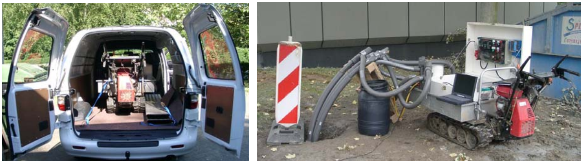
Figure 4: Latest generation of UbeG test units (GeRT); transported to the site in a small van (left) and moved on site to the BHE on a crawler, even in rough terrain (right)
