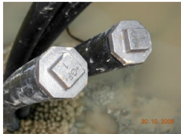
Figure 14: Sealing the BHE's
