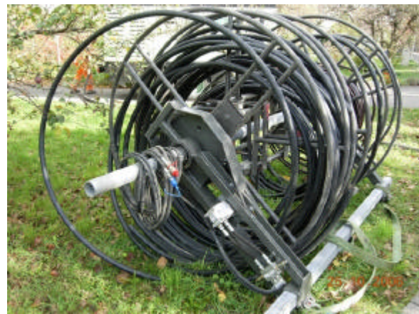
Figure 13: Preparing the BHE on a decoiler with hydraulic brake
