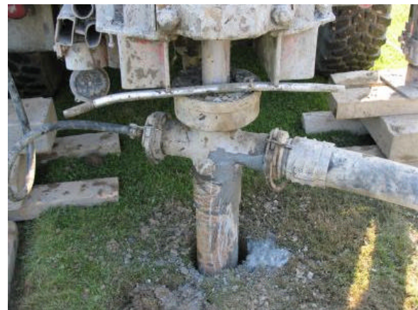
Figure 11: Drilling equipment with preventer and dense water/mud management
