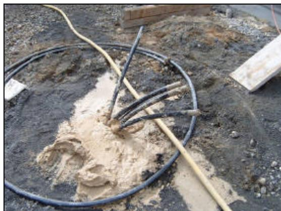
**Figure 5: View of a grouted double-U BHE top**
