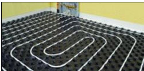
Figure 10: Floor heating system.
