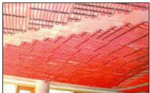
Figure 12: Ceiling cooling system.
