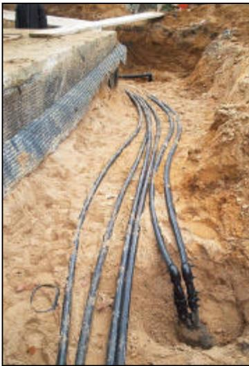
**Figure 7: Piping connecting BHEs to the manifold**
