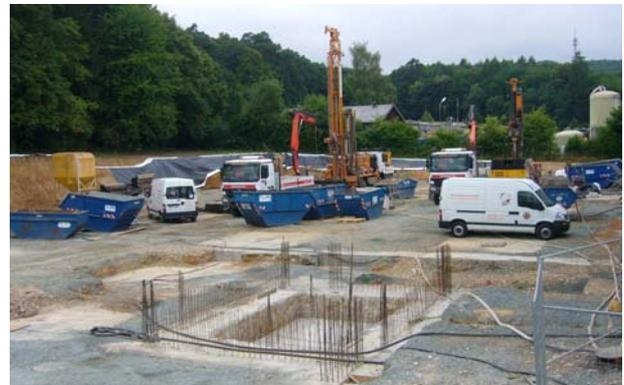
**Figure 7: Drilling of 250-m-boreholes from the planum of the construction pit for the new building, 2008**
