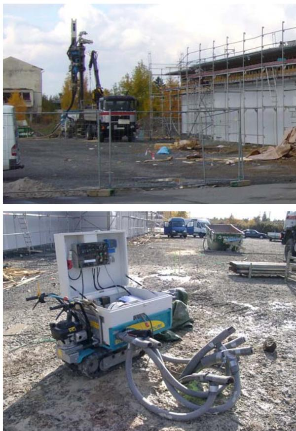
**Figure 3: Drilling for BHE on supermarket construction site (top) and TRT on the same site (bottom), 2008**
