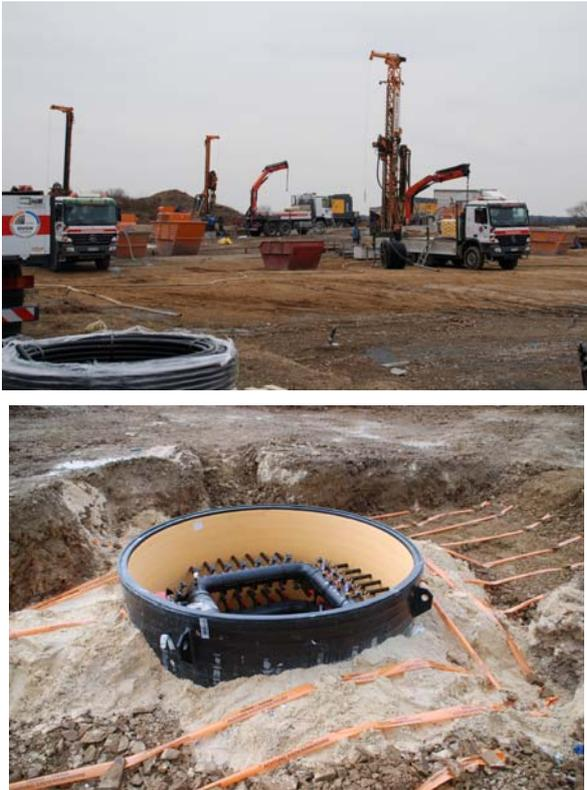
**Figure 16: Drilling for Leica BHE field with 3 rigs in parallel, February 2012 (top) and manifold for the field with 50 BHE (bottom)**
