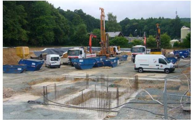
**Figure 7: Drilling of 250-m-boreholes from the planum of the construction pit for the new building, 2008**
