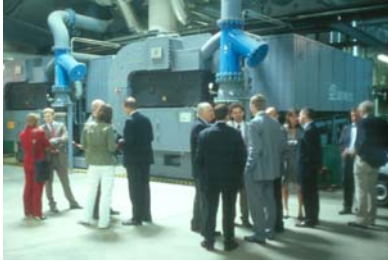
Absorption Chiller (example Barcelona, driven by waste heat from waste incineration)
