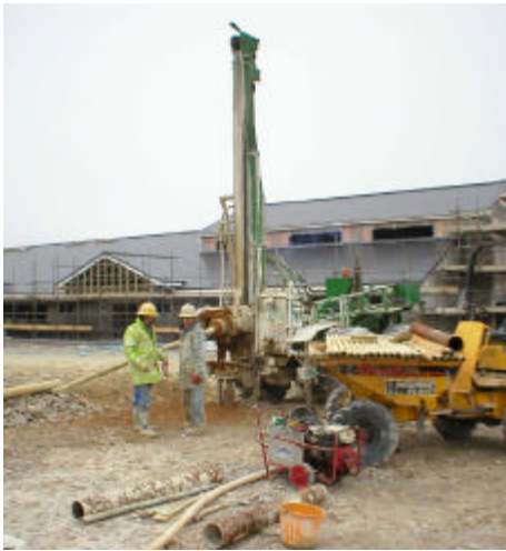
Photo 3. Drilling for a GSHP installation in progress in Cornwall, UK (Geoscience).
