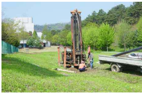
Figure 3: Drilling on the KEPRI site in April 2003 (photo Choi)
