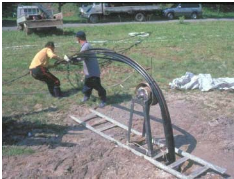
Figure 4: BHE pipe installation in April 2003 using a makeshift roller device (photo Sanner)
